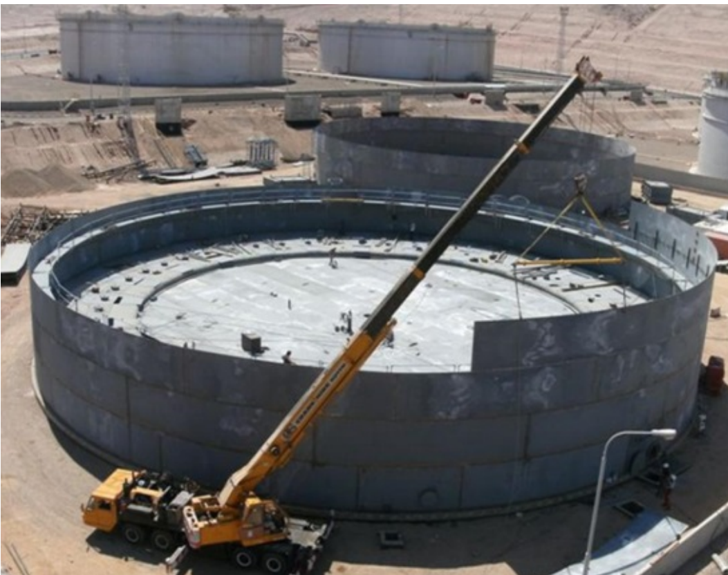
Inset 4.35: Example storage tank under construction (larger than the proposed)
