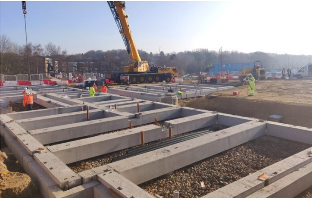
Inset 4.13: Example of precast ground beams
