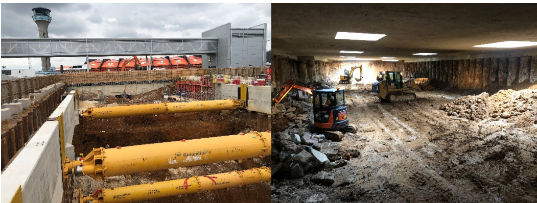
Inset 4.24: Open box and top-down construction on Luton DART scheme
